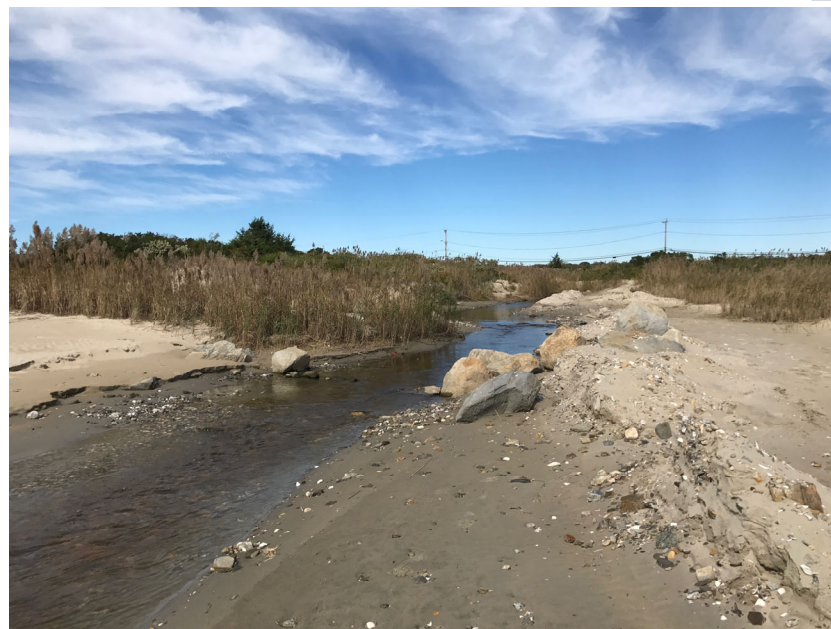
10) October 16, 2018. Outlet Channel (Beach Side)
