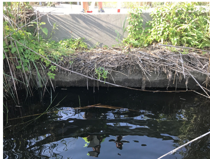
6) August 07, 2018 Concrete box culvert (Pond Side)
