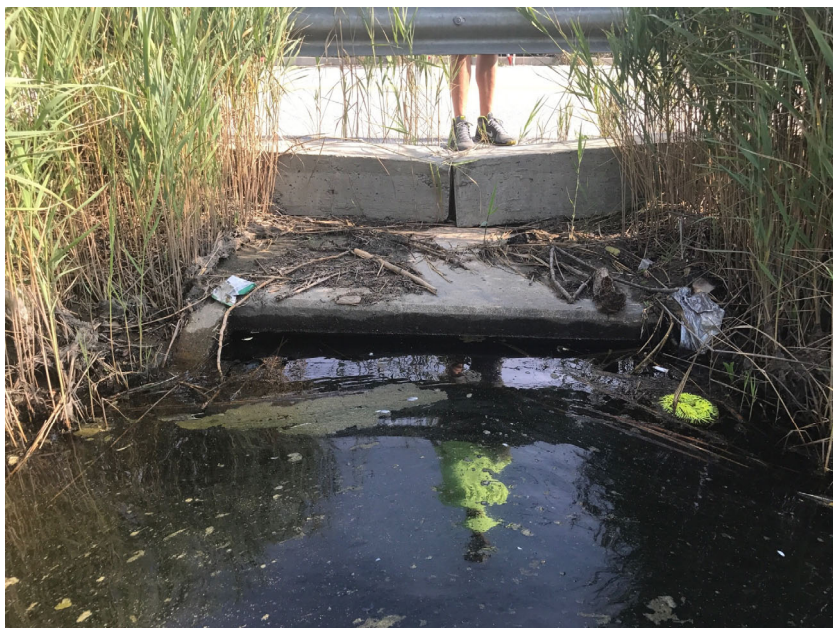
7) August 07, 2018 Concrete box culvert (Beach Side).
